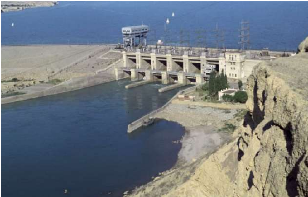
Fig.1. General view of Talimarjon Reservoir
