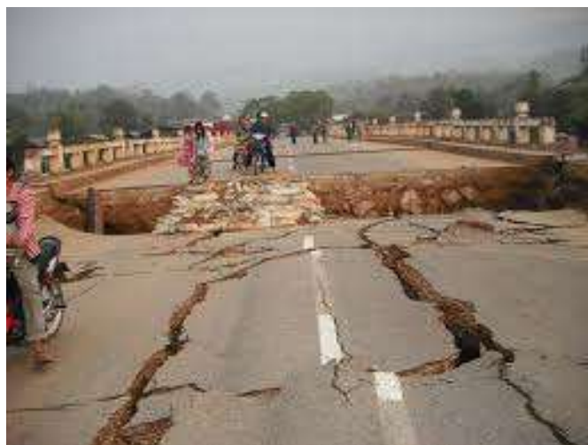
Figure 1. Ground displacements in Burma earthquake (adapted from Ref. [1])
